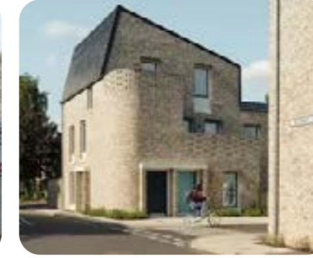
Goldsmith Street, Norwich Built to Passivhaus standards, needing little energy for heating and cooling.
