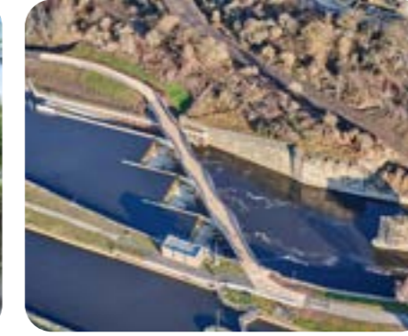
Knostrup Weir, Leeds | Flood Management Provides three new pneumatically moveable weirs that can be lowered to let floodwater discharge quickly downstream.
