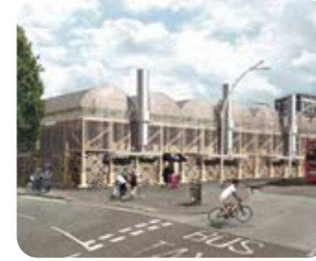
Illford Community Market, London Designed for five year and will be dismantled and reconfigured on future meanwhile sites.
