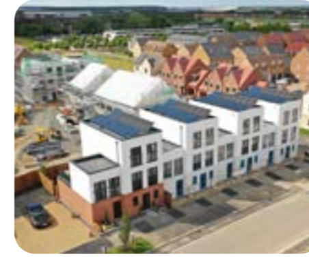
Project Etopia, Corby Uses combined solar PV's and thermal panel to deliver net zero carbon on site.
