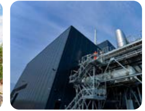
Millerhill, Midlothian Residual waste recycling and energy recovery facility
